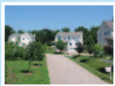
Individual homes at Jordan Cove have pervious driveway materials, rain gardens handling roof runoff, and “no mow” zones in the back yards featuring native vegetation. A sunken, vegetated cul-de-sac center accepts and treats runoff and there are swales located on each side of the street.
